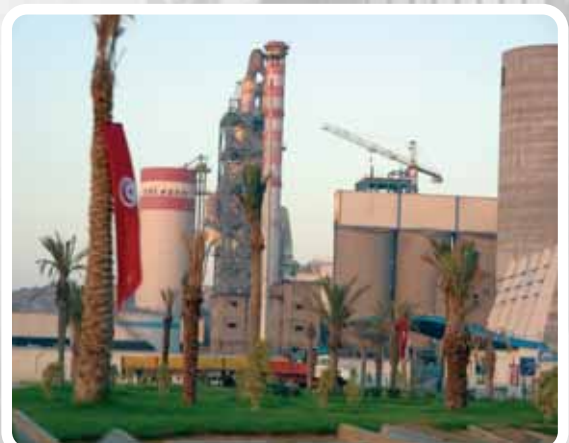
Cimenterie Cement plant
