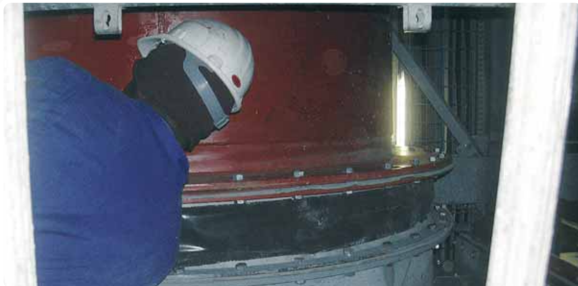
Montage compensateur en UIOM sortie Electrofiltre - Temp. 250°C Mounting of a Household Refuse Incinerator compensator Electrofilter exit - Temp. 250°C
