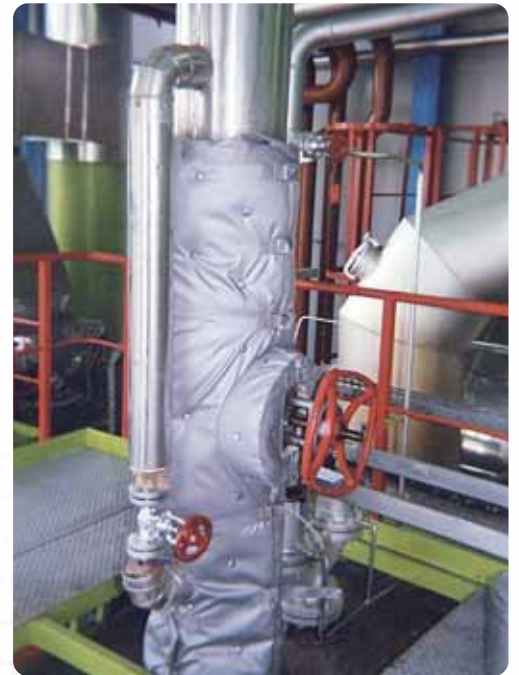
Matelas de vanne - Isolation 600°C Valve stuffing mats - 600°C Isolation
