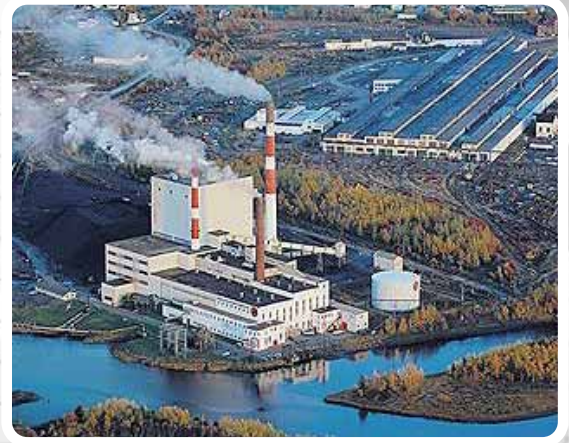
Centrale thermique Thermal Power Station
